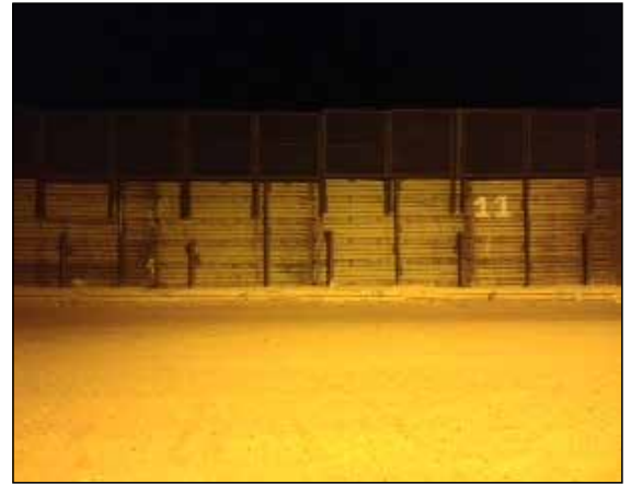
Douglas/Naco Border Fence as we saw it on Feb. 9, 2013
